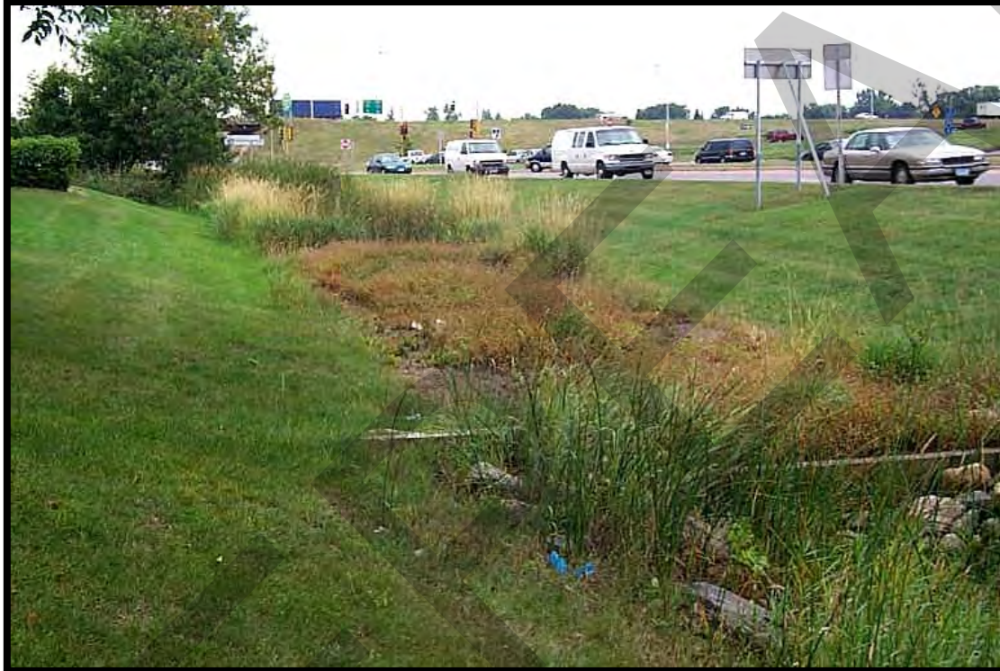
Figure C-3 Wet Swale Used to Treat Highway Runoff
